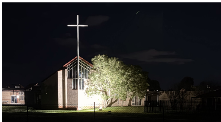
The new lighting on Holy Family Church
